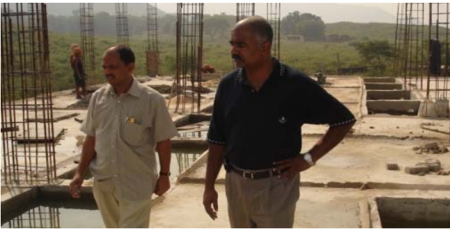
Mark Paul, Consultant DIK-Germany, with the Director KEHRC at the construction site of New KEHRC
